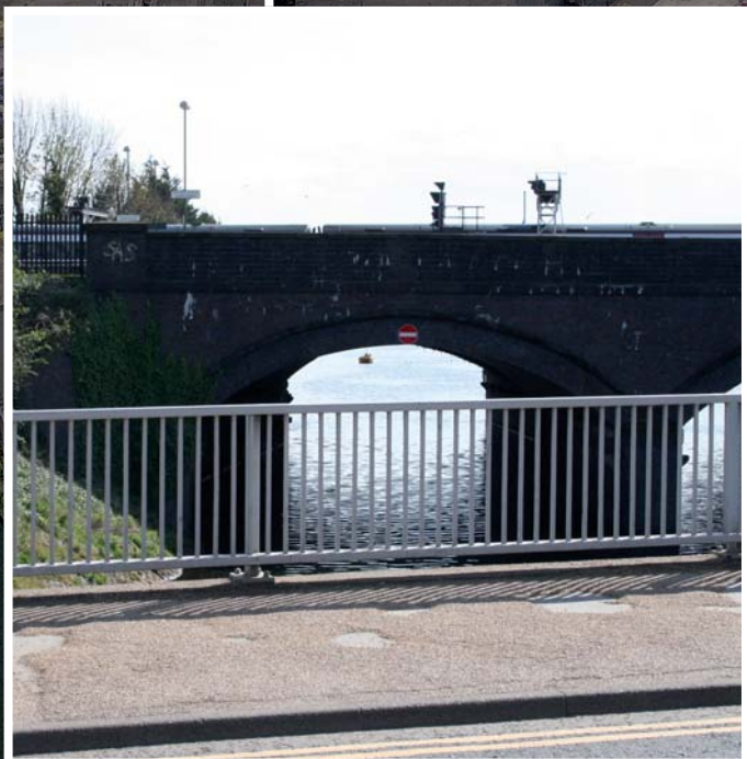
RIVERFRONT WALK DISCONNECTED
