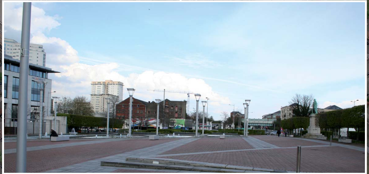
CALLAGHAN SQUARE LACKS ACTIVE FRONTAGE AND FOOTFALL
