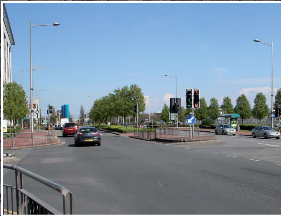
ROADS DOMINATE THE SPACE
